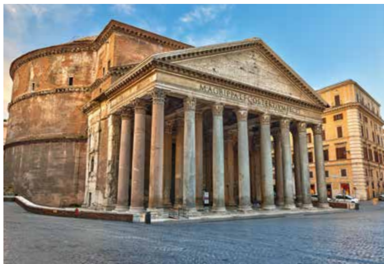
The Pantheon in Rome, built in 27 B.C., is the largest construction ever built out of non-reinforced concrete.
