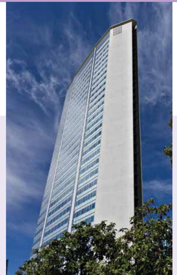
The Pirelli Tower in Milan, designed by Gio Ponti in 1950 and built by using reinforced concrete.
