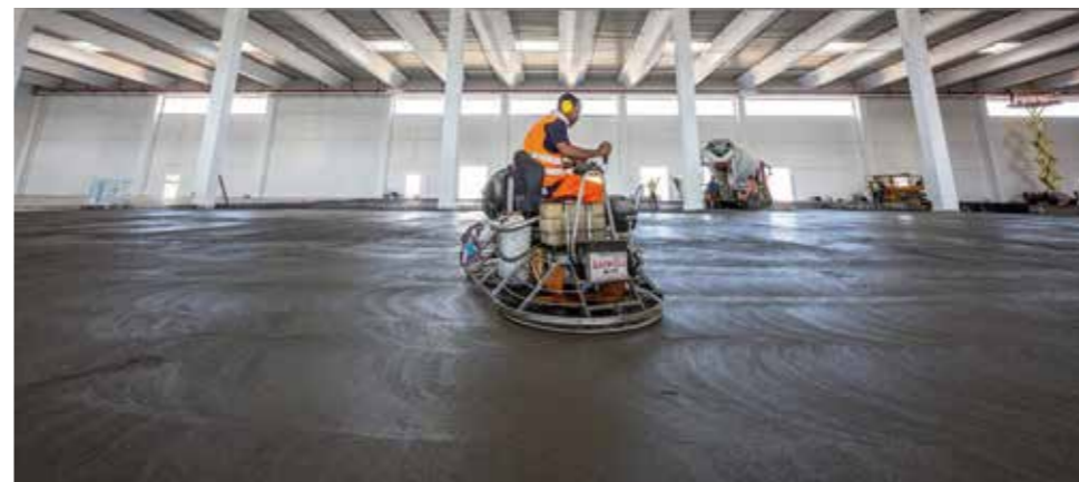
LEFT. The extrusion process is used to produce synthetic fibers at the Mapei manufacturing facility in San Cesario Sul Panaro in the Province of Modena (Italy). RIGHT and BELOW. An example of concrete industrial flooring strengthened with synthetic fibers for the Docks logistic centre in Serravalle Scrivia (Italy).
