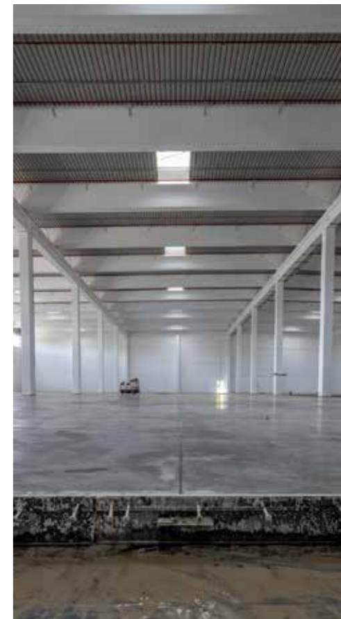
LEFT. The extrusion process is used to produce synthetic fibers at the Mapei manufacturing facility in San Cesario Sul Panaro in the Province of Modena (Italy). RIGHT and BELOW. An example of concrete industrial flooring strengthened with synthetic fibers for the Docks logistic centre in Serravalle Scrivia (Italy).
