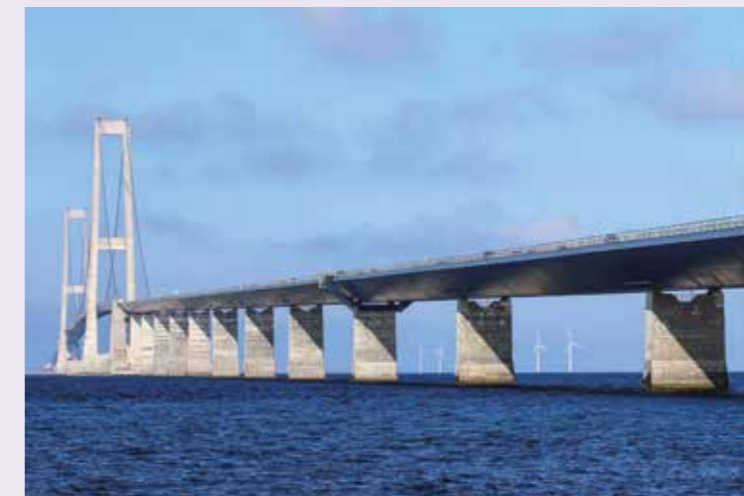
Concrete structures perform excellent durability, such as the Storebælt Bridge in Denmark.
