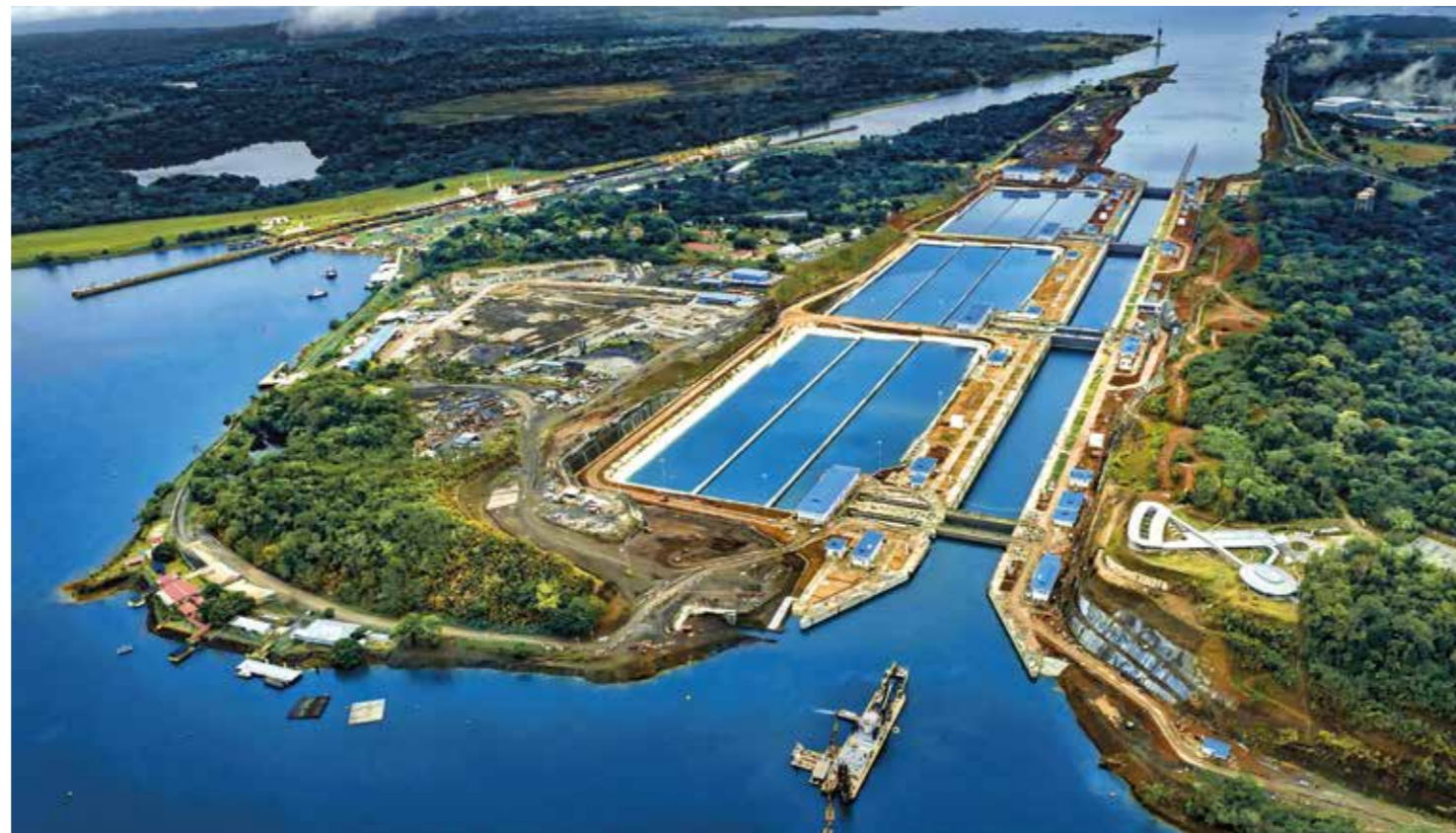
The Panama Canal: an imposing project for which Mapei supplied admixtures (such as DYNAMON XP2 and DYNAMON XP2 EVOLUTION) to reduce the water/cement ratio and increase the durability of concrete. This contributed to its estimated design life of 150 years.
