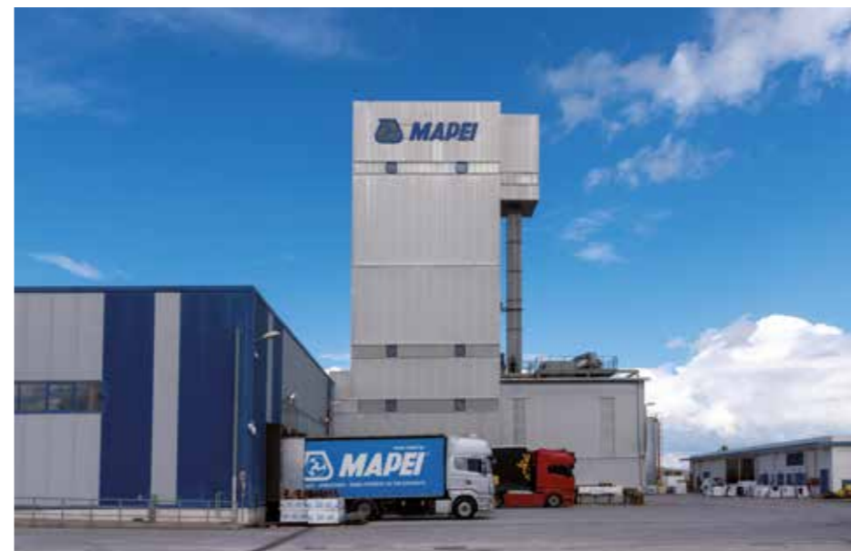
Mapei Hellas' plant is located in Ritsona, not far from Athens.
