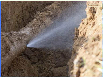
Source: https://shorturl.at/mV6ED Fig. 7 Underground Leak
