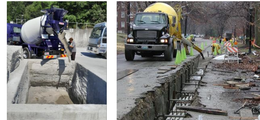
Fig. 3 RC and utility backfilling (NRMCA)
